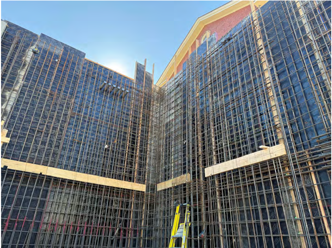
High wall rebar installation, 0826
